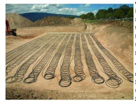
cooling) from the earth for use indoors. This is done by running heat transfer fluid through thermally conductive pipe. The fluid stays in the pipe at all times and only heat is absorbed from the earth.
